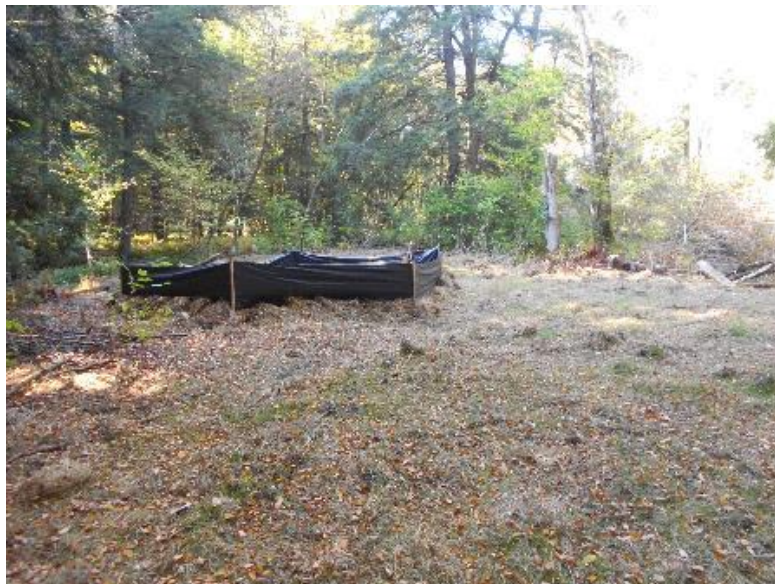
Biopod delineated by silt fence and “confluence” area seeded and mulched.
