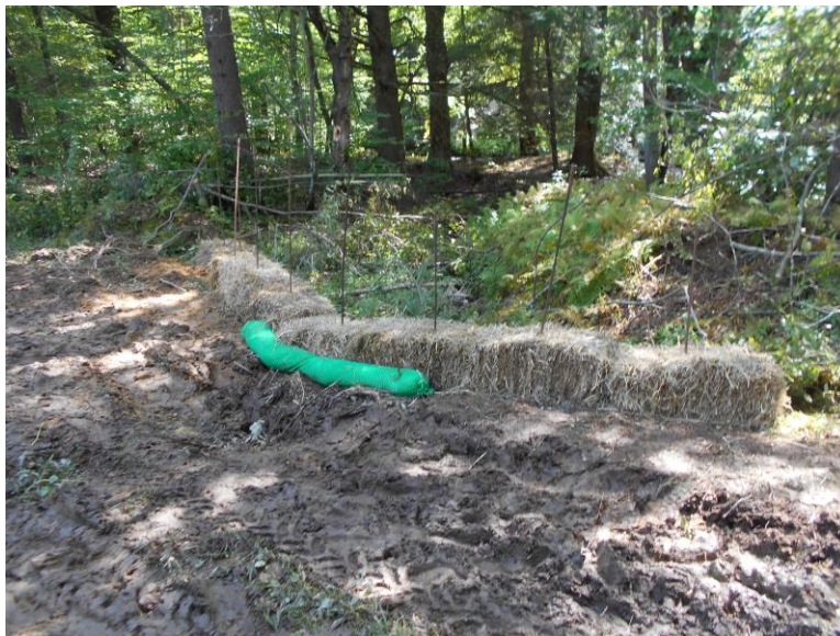
Access Road E &S measures.
