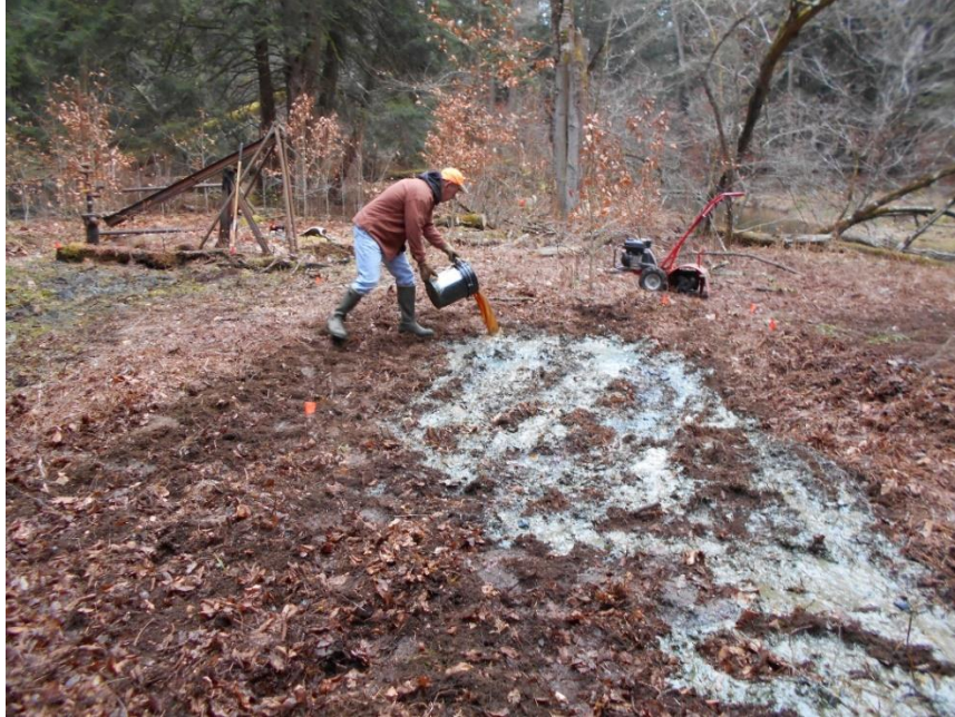
Crude oil collected from the abandoned well spill is poured on the ground and cultivated into the soil to create the biopod where microbes digest the oil.
