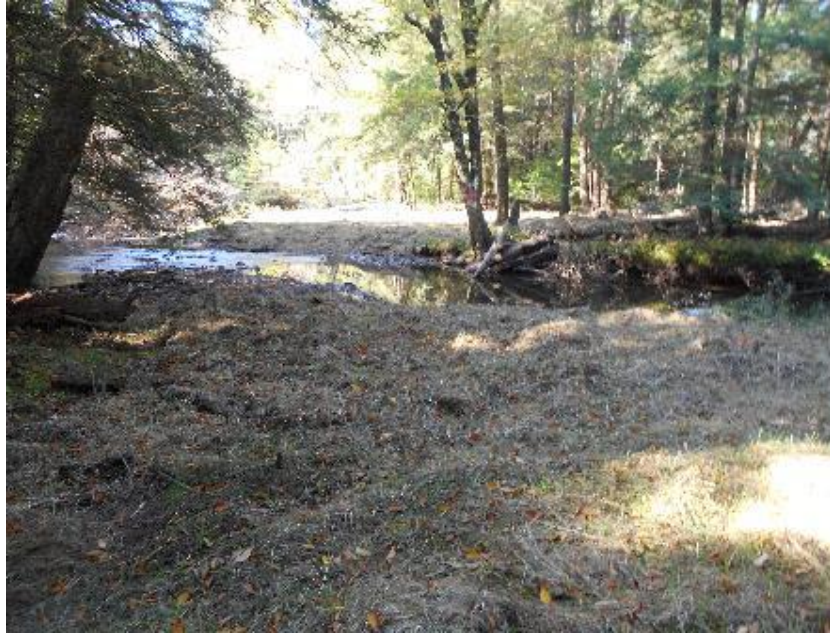
Stream crossing restored, seeded and mulched.
